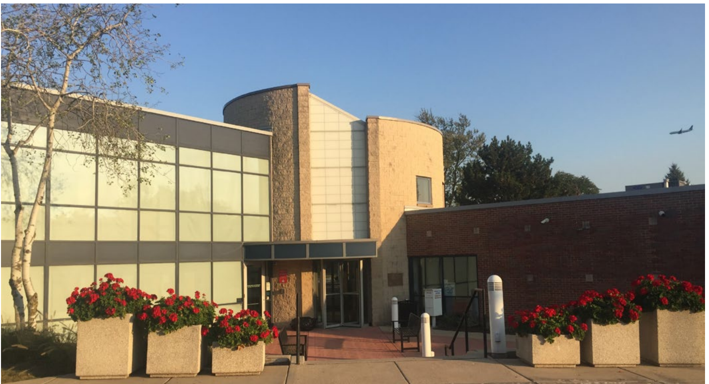
Wood Dale City Hall
